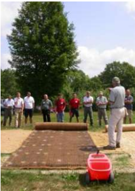
Participants learn how to install an erosion control blankets at the District's Field Day.
